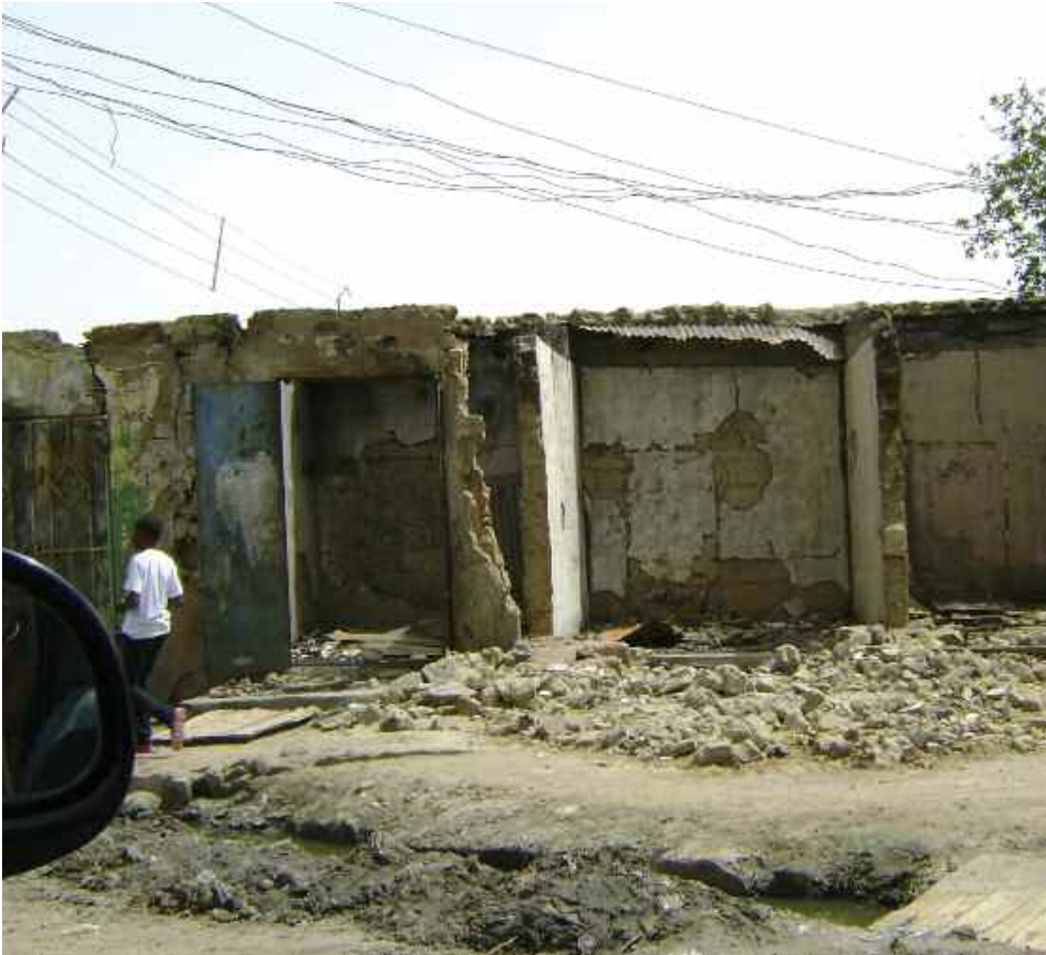
Above and above right: Shops and houses allegedly burnt by the Joint Task Force (JTF) at Lawan Bukar junction, Maiduguri, on 22 May 2012. After Ibrahim Bukar Tela locked himself in his shop (above) for protection, JTF members reportedly set it on fire, killing him.
