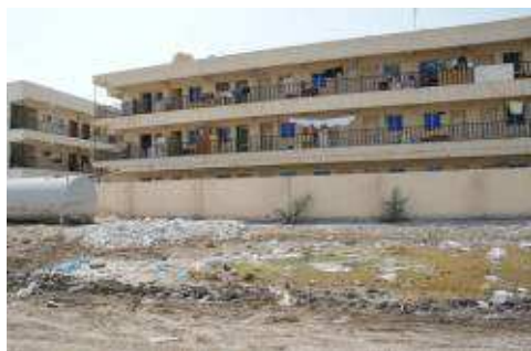
Sewage overflows in the street. Doha's Industrial Area, October 2012 © Amnesty International
