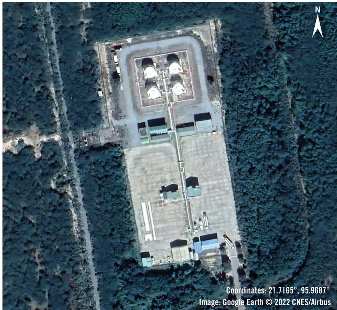
NEPAS storage facility at Mandalay airport.
