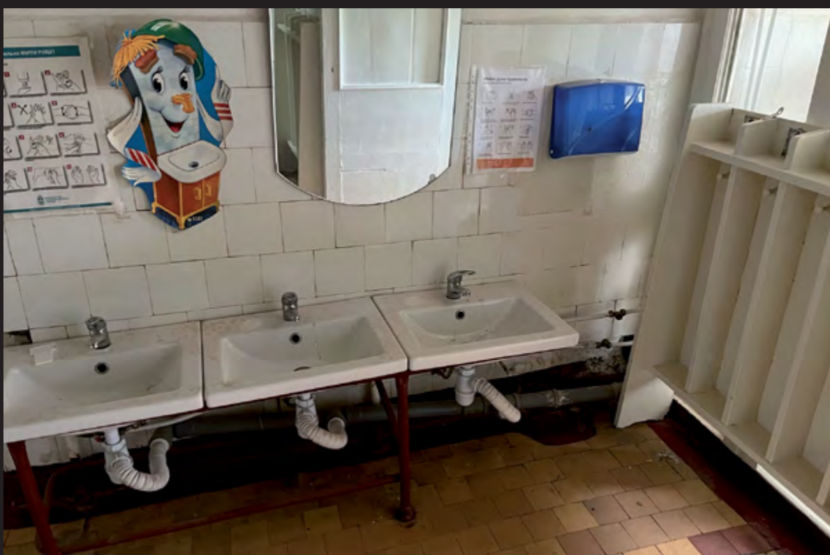
↑ A bathroom facility in a temporary shelters for displaced people in Kharkiv, Ukraine. Shelters, which are often in schools or nurseries, often do not have physically accessible sanitation for people with disabilities. © Amnesty International
