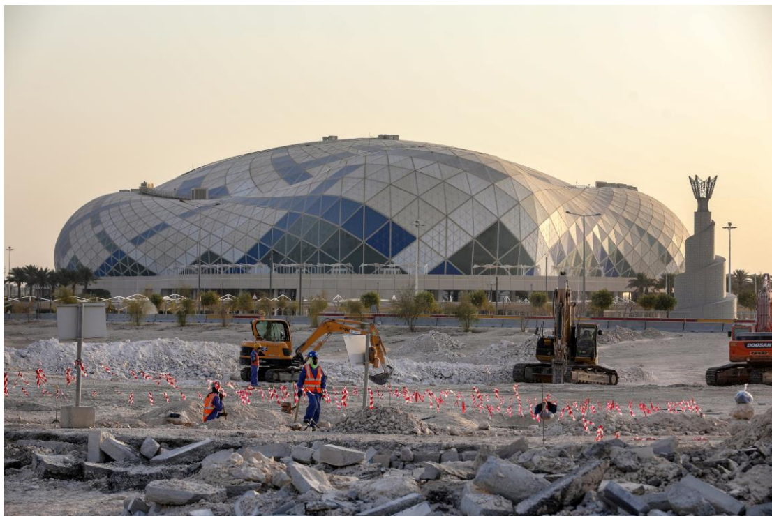
Workers seen at the construction site of Lusail Stadium, a venue for 2022 FIFA World Cup football matches. © Valery Sharifulin/TASS
