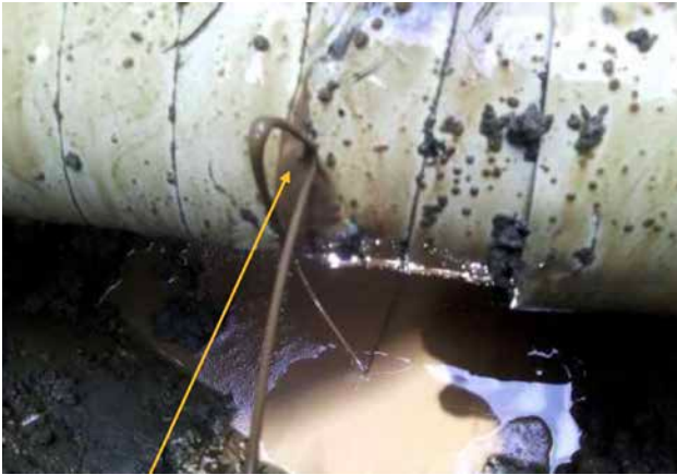
Spill on Shell's "4" Obele-Ibaa Delivery Line" at Ibaa/Omueze, 2015. Shell photograph.
