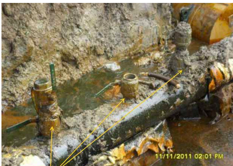
Oil theft points on Shell's 12" Imo River - Ogale pipeline on 13 November 2011. Shell photograph.
