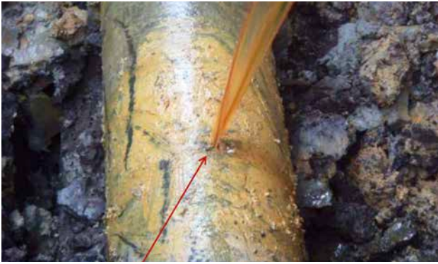
Leak point at Shell's 10" Diebu Creek-Nun River pipeline at Onyoma (2014) . Shell photograph.
