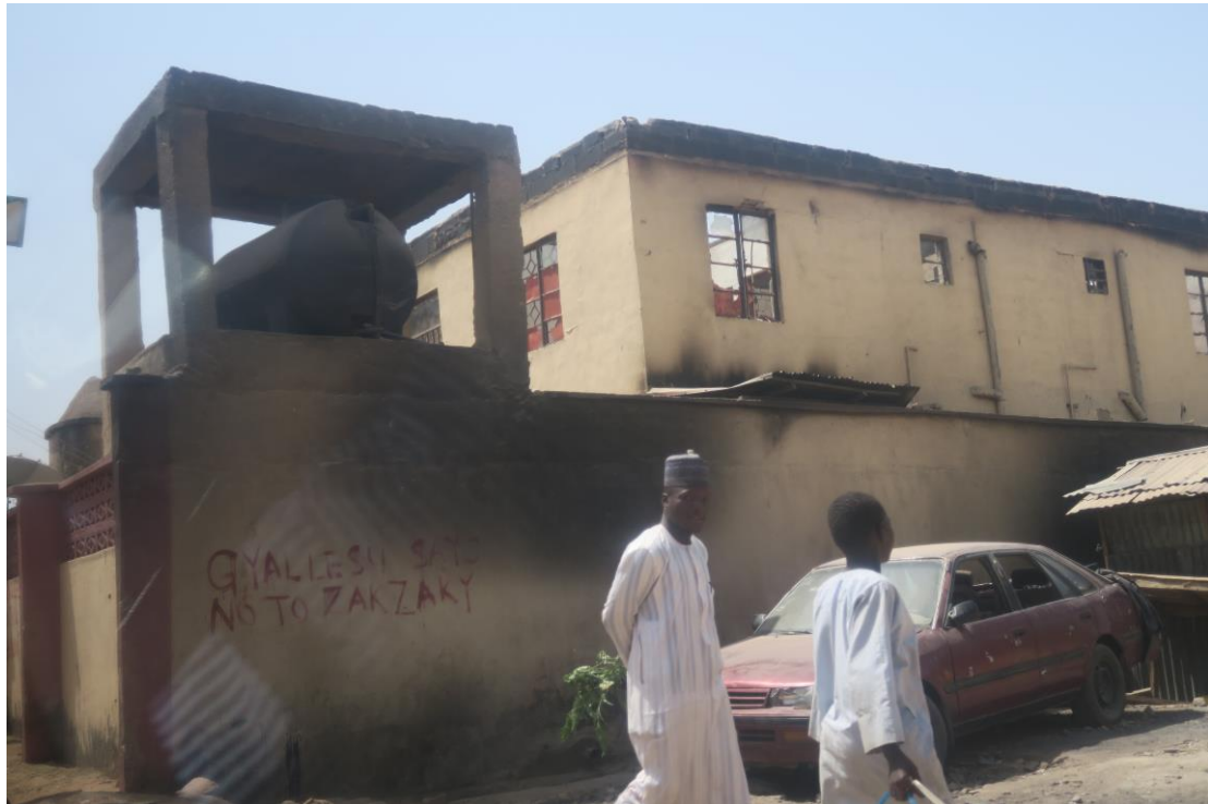
Anti Zakzaky graffiti on burned down building in Gyallesu neighbourhood, Zaria © Amnesty International
