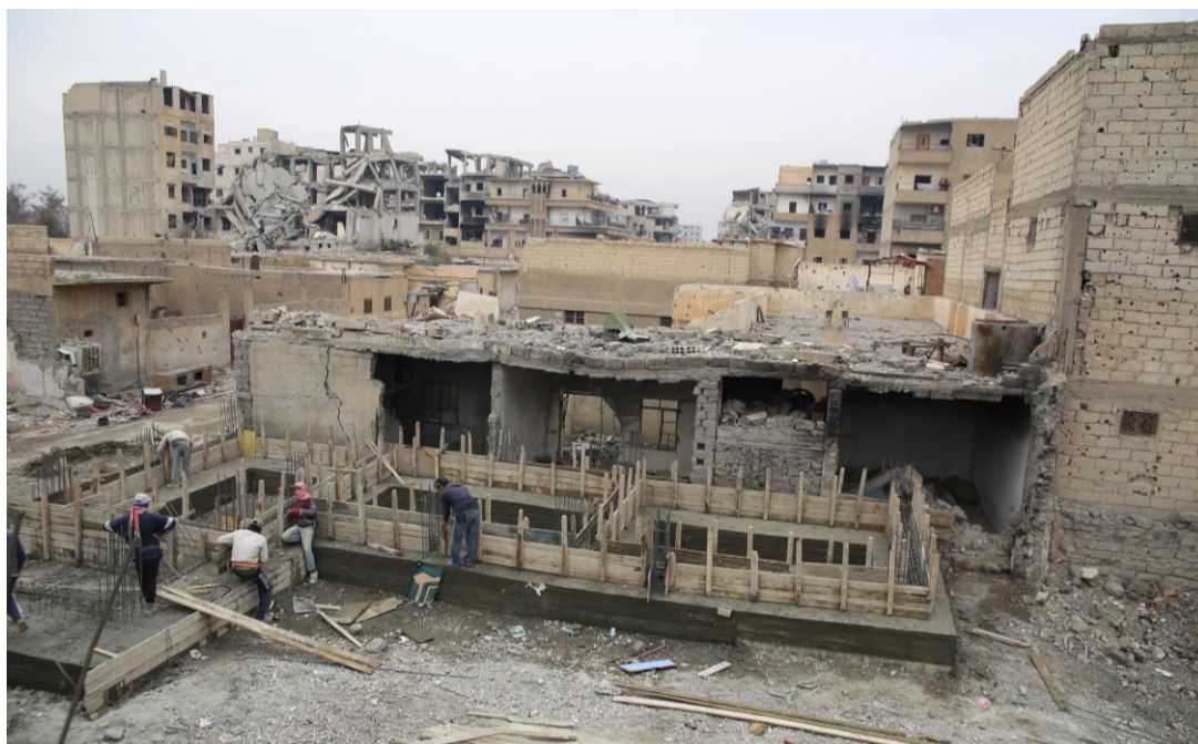
Workmen are rebuilding the Fayad family home, which was destroyed in a Coalition air strike on 12 October 2017 in Raqqa. © Amnesty International
